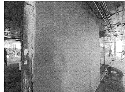
Plaster work for shear wall & column
